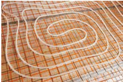
Floor heating loop
